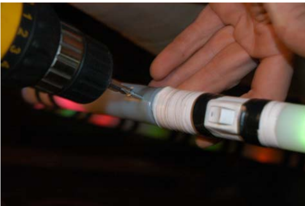
Figs. 8-9 If the fit seems a bit loose (re-heating can sometimes do this), we recommend drilling a small hole and fitting the connection with a screw.
