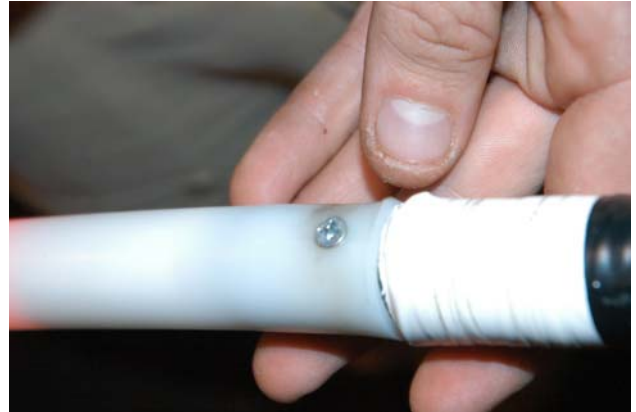
Figs. 8-9 If the fit seems a bit loose (re-heating can sometimes do this), we recommend drilling a small hole and fitting the connection with a screw.
