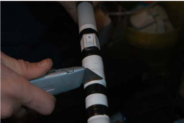
Fig. 1 Cut the tape at the connector.
