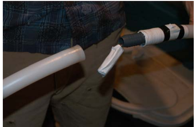
Fig. 4 HEAT the end of the pipe using a lighter, hair dryer, or other heat source. Pull open the connector. If the pipe does not open easily, continue heating.
